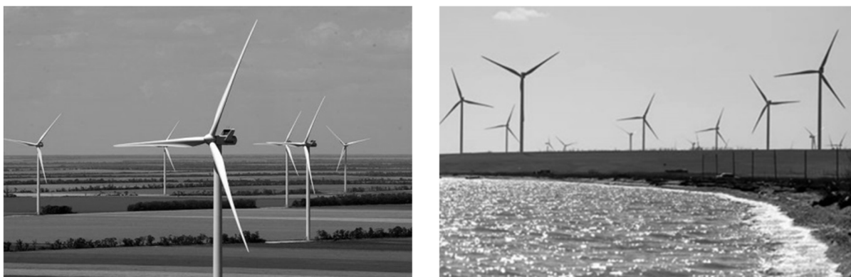
Fig. 3. Wind Turbines of Botiev Wind Plant
