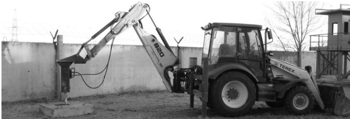
Fig. 5. Installation of concrete breaker and the creation of dynamic impact
