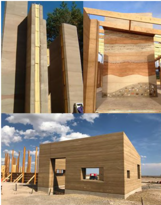
Fig. 4.12. Soil concrete buildings [18, 19]
