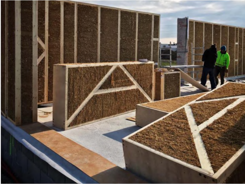
Fig. 4.6. Prefabricated straw bale wall panels [15]
