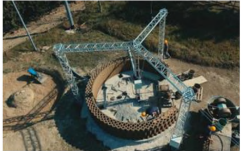
Fig. 6.9. Italy, Gaia House, 2018, Dwelling house (natural mixtures from the soil of the adjacent territory, waste from rice production, crushed straw)
