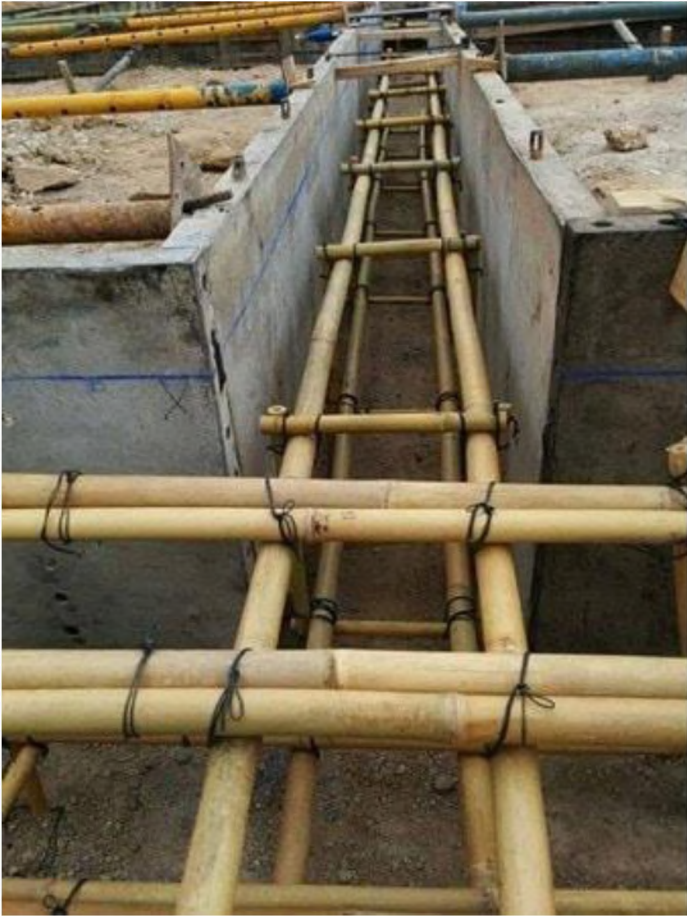
Fig. 4.15. Foundation reinforcement with bamboo rods [20]
