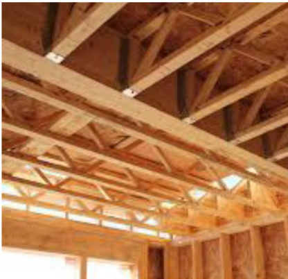
light weight trusses
