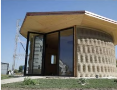
Fig. 6.9. Italy, Gaia House, 2018, Dwelling house (natural mixtures from the soil of the adjacent territory, waste from rice production, crushed straw)
