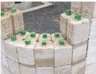
Wall of Hempcrete lego-block [10]
