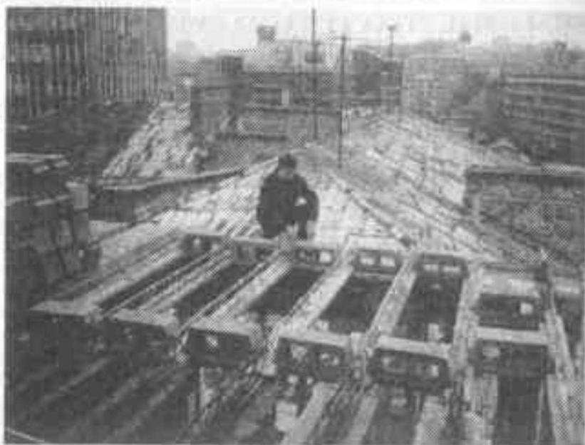
Figure 1: Reconstruction building from small size structural elements, Dnipropetrovs'k
