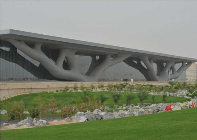
Figure 2. Educational center, Doha, Qatar
