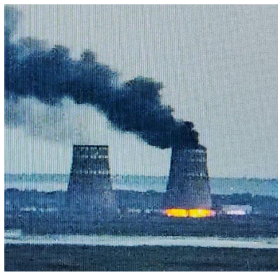
Fig. 2. Fire at the cooling tower of Zaporizhzhia NPP in 2024
