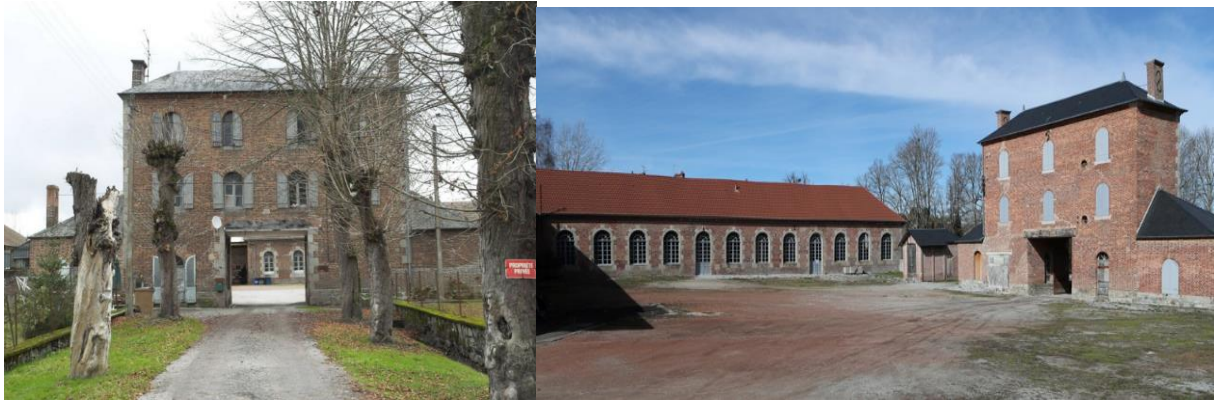
Fig. 4. Mine equipment and tool repair workshops
