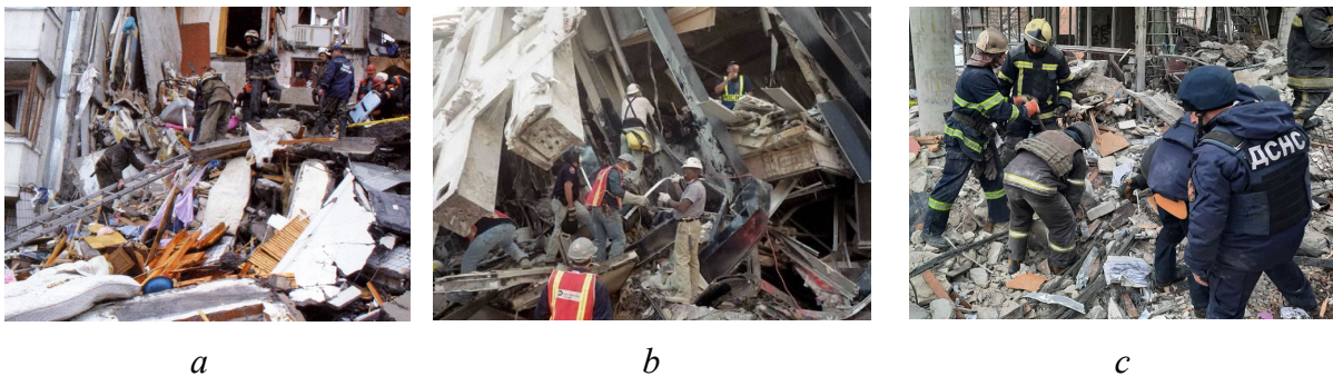
Fig. 1. Determination of the nature of structural damage by visual inspection: a – Dnipro (2007); b – New York (2001); c – a – Kharkiv (2022)
