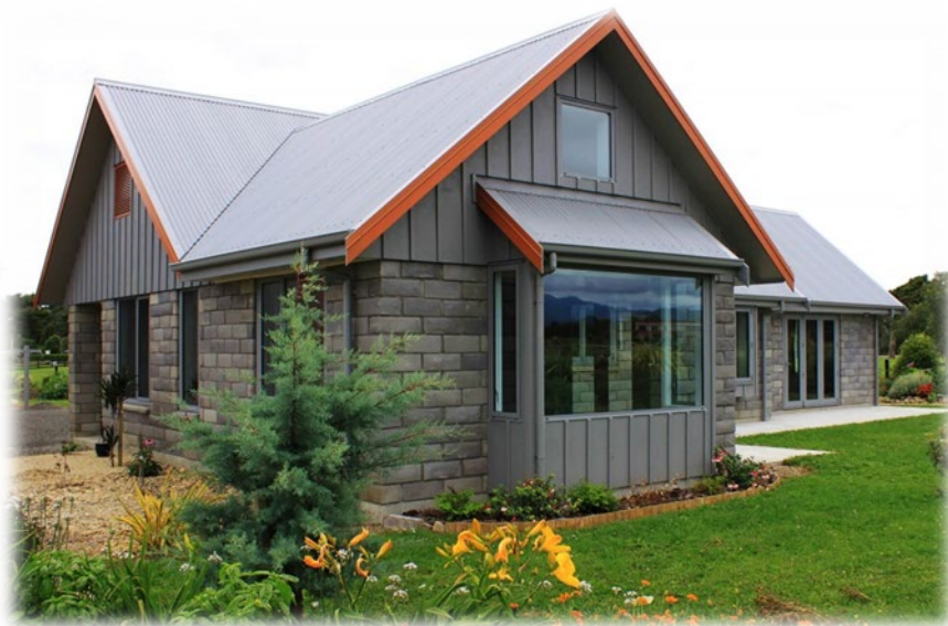
Fig. Examples of buildings with structures made of ecological concrete
